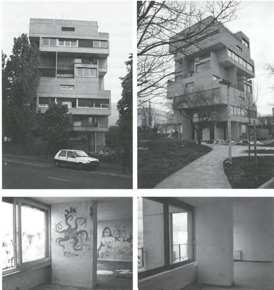
FIGURE 4. Atelier de Montrouge , EDF staff housing towers, Ivry-sur-Seine, 1963-67. Photographic report 2002; 2016. © Catherine Blain.
